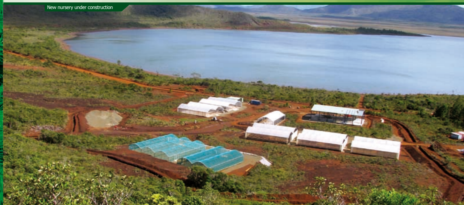
New nursery under construction
